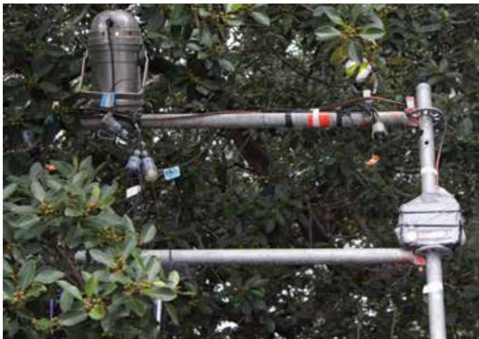
Zactrack anchor rigged at the rear of the seating area ▼
